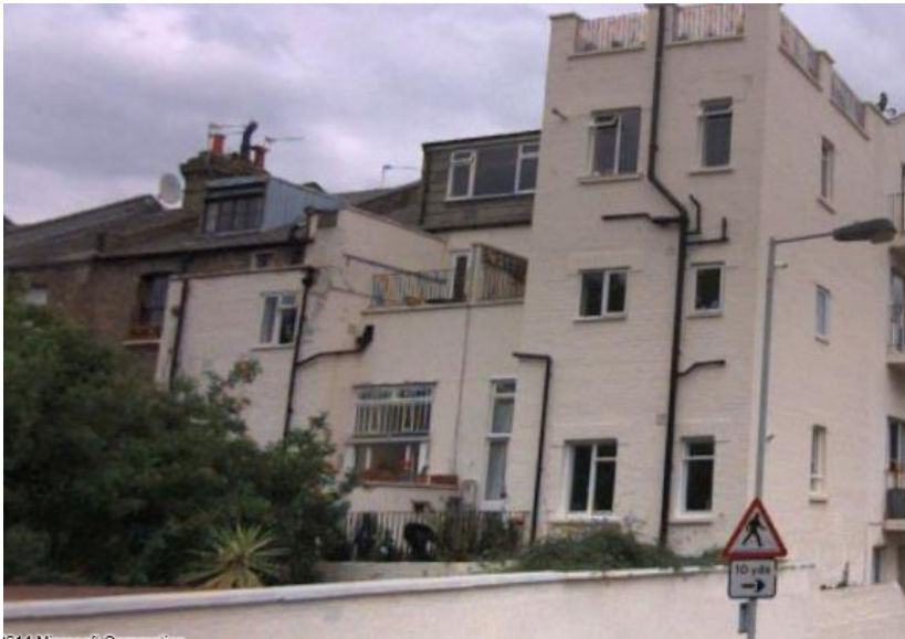
Image 2: Rear of the building viewed from Cardozo Road
