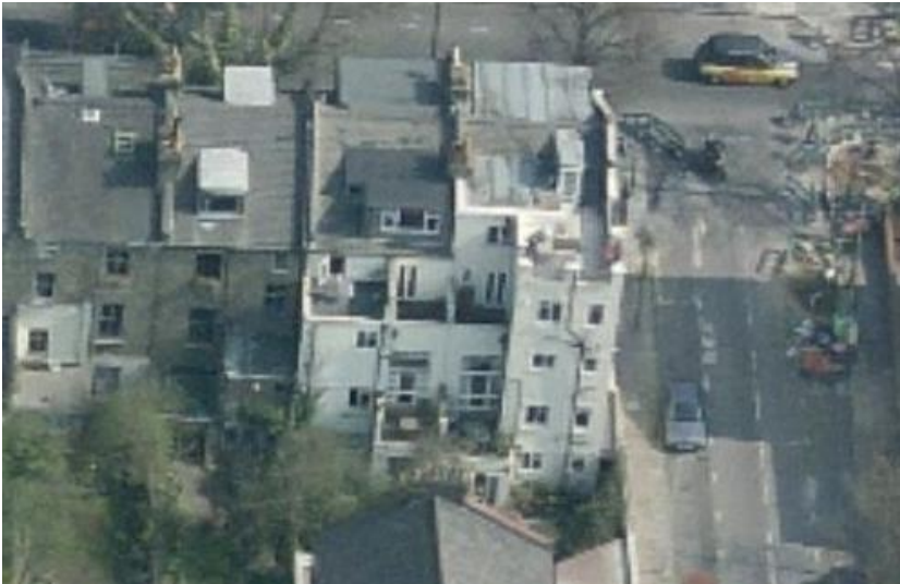
Image 1: Aerial photograph showing the rear elevation
